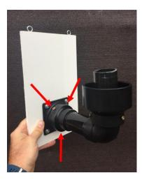
Seal the bottom of the moat with silicone sealant and fill tube with spray foam, trim off spray foam at the top of the pipe stand when dry. Allow plenty of time (like, several days) for silicone sealant to dry.
